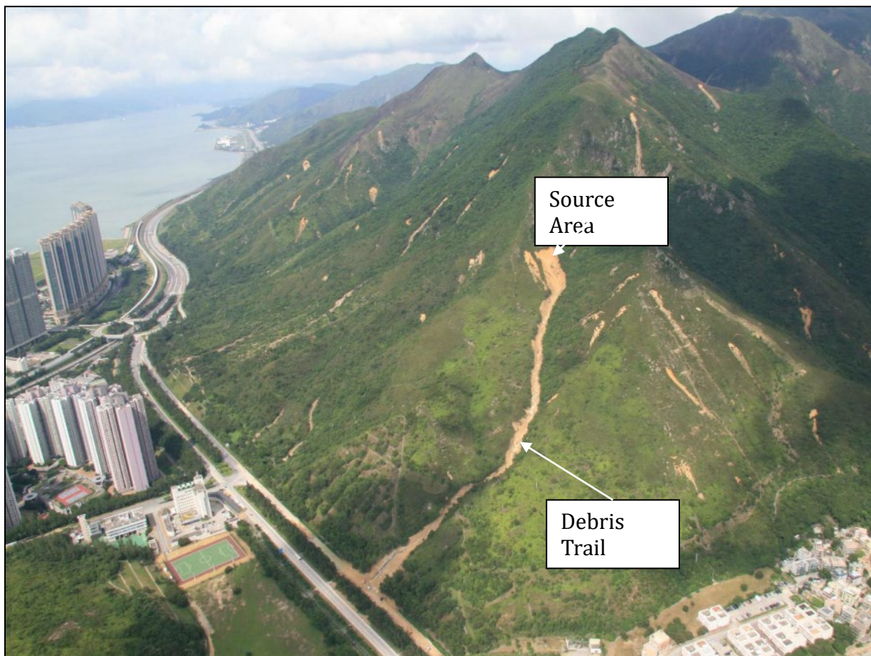
Figure 3– Large CDF generated by the June 7 2008 Rainstorm at Yu Tung Road, North Lantau.
